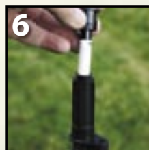
6 Install MP Rotator
